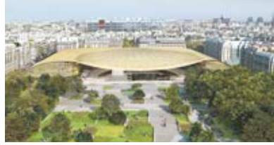
Le Forum des Halles Paris, France (extension-renovation) +15,049m 2 GLA Complete refurbishment and extension of a Paris landmark.
