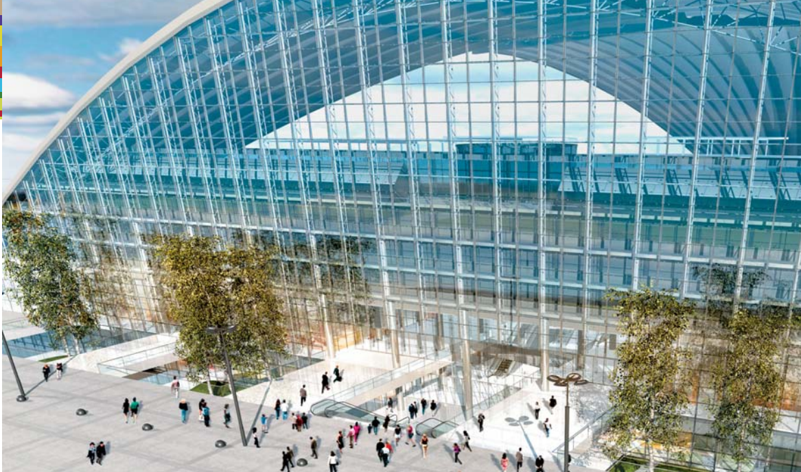
CNIT: redevelopment of an iconic building at La Défense.
