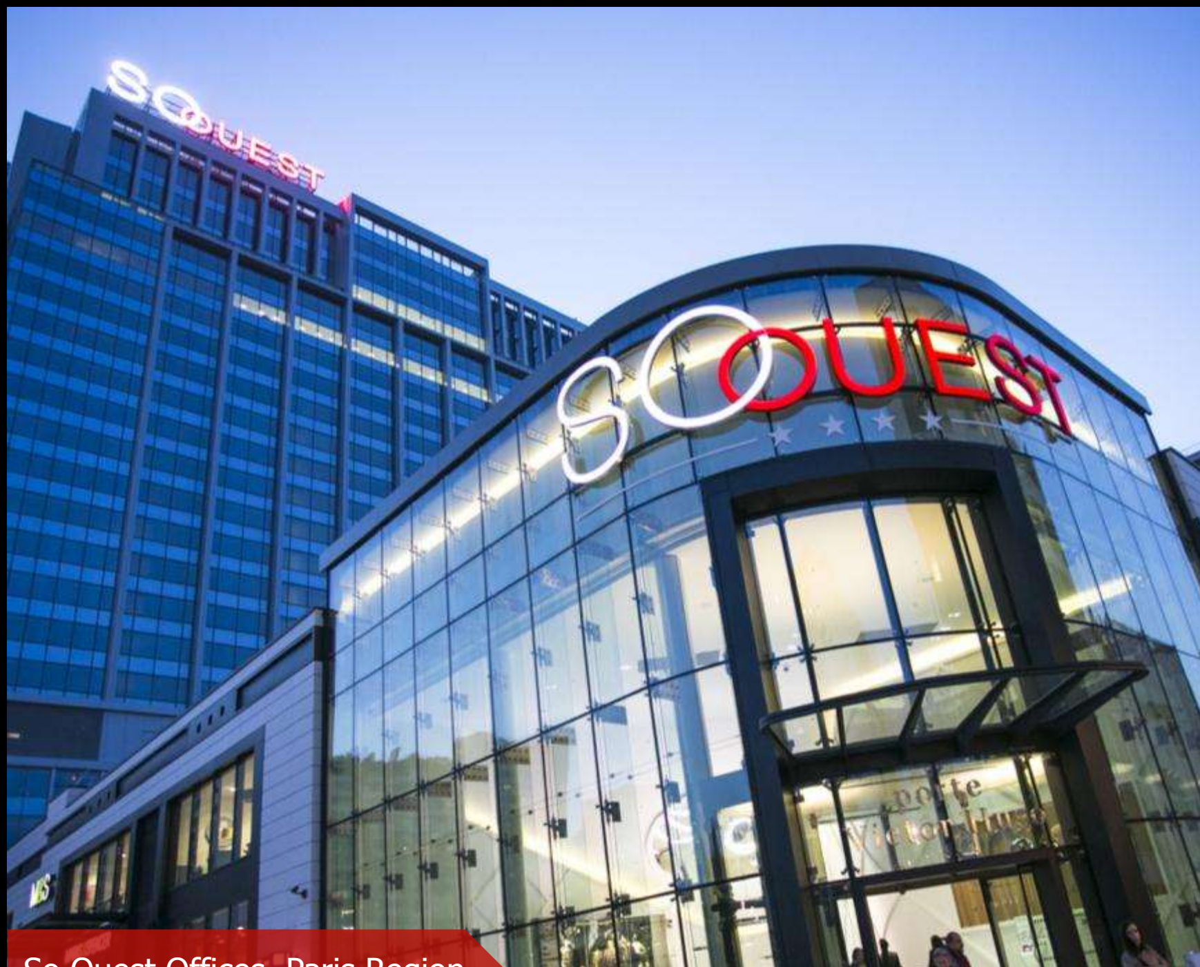
So Ouest Offices, Paris Region
