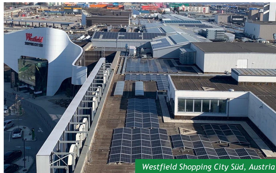
Largest solar PV system on a shopping centre in Europe
